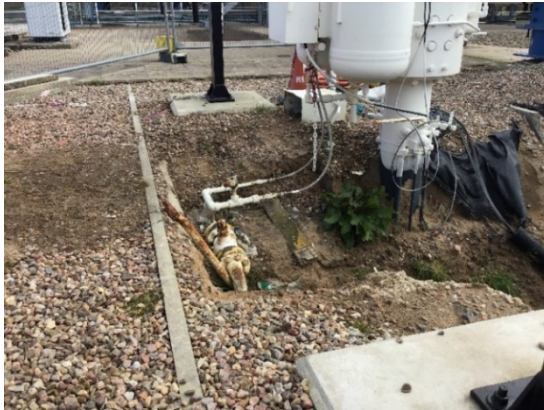
Figure 44: Corrosion and ground movement threats to Actuators
